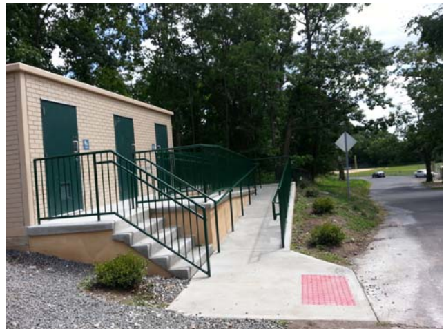
Prospect Park – Hofstra Park Bathroom construction
